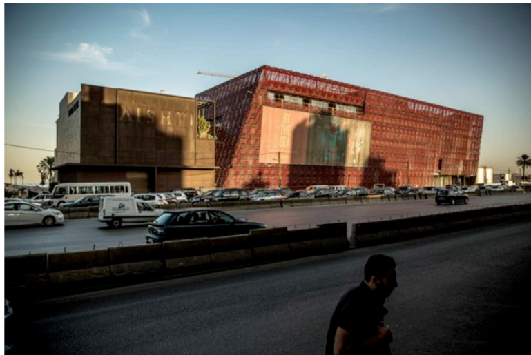
The Aishti Foundation, which shares a building with a large retail space for luxury brands, was designed by the architect David Adjaye. Bryan Denton for The New York Times
